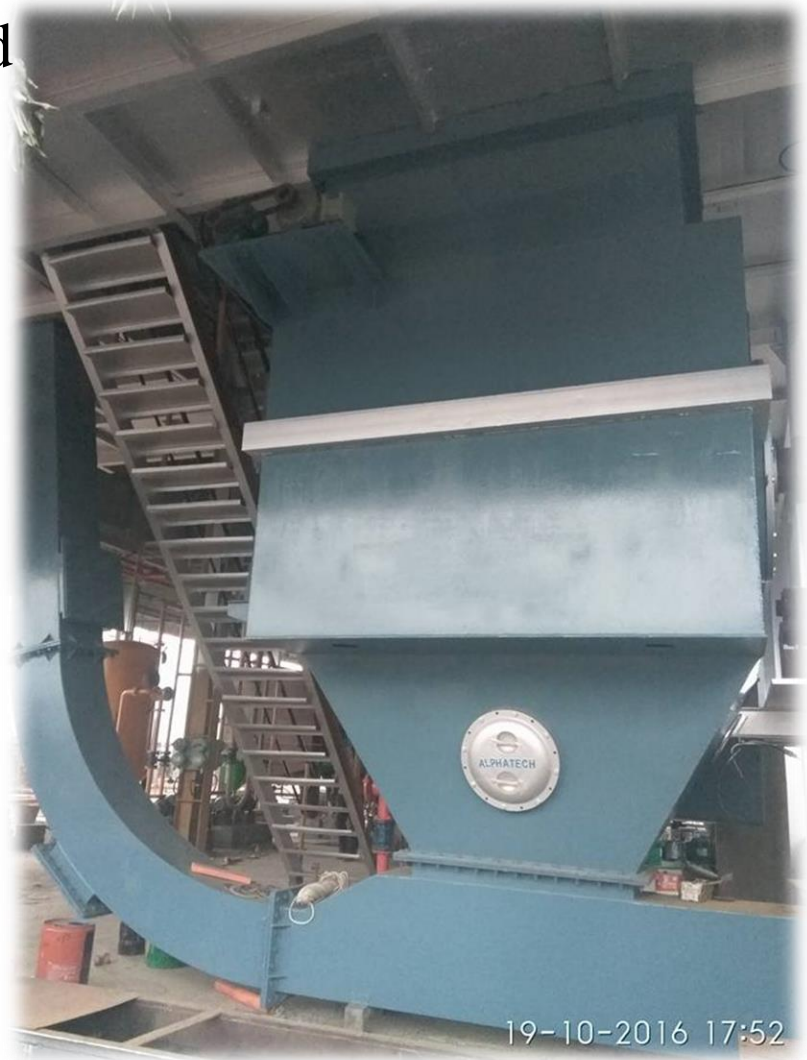
200 tonnes per day capacity CSM solvent extraction plant at Mallepalli, Telangana State
