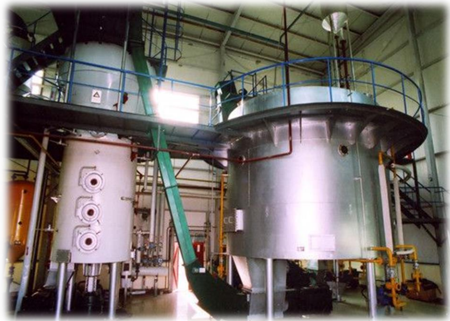
Pre-press solvent extraction unit
