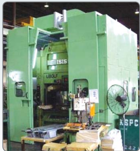
Actual Installation of Acoustic Enclosure at Site
