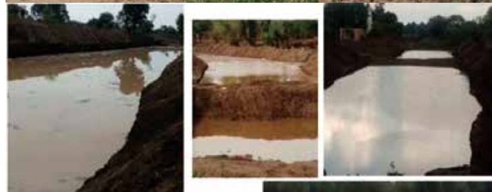
Before-After Excavation & Post Rain in Paradh Village in Bhokardan Talukas
