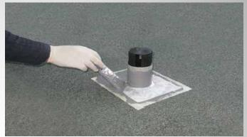
**Pipe Penetration** Seal the gap between pipe and slab using TOBSLAK ATU FAST 100 for about 2 inches in diameter.
