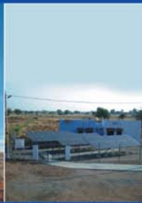
Off Grid System
