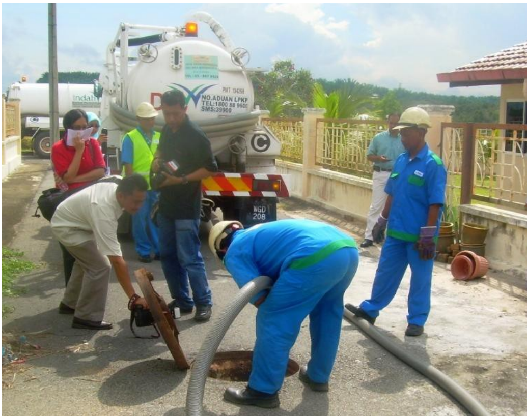
IWK network crew clearing hardened sludge from abandoned sewer at Taman Impian Jaya, Senai, Johor.
