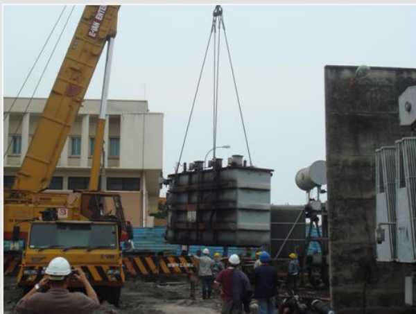
Figure 11: Discarded Transformer from the Switchyard
