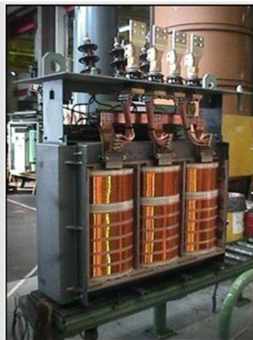
Figure 13: Copper Coils Within a Transformer (Source: Copper Alliance UK)
