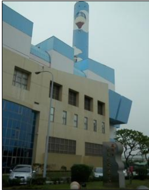
Figure 23: Renwu Waste Management Plant
