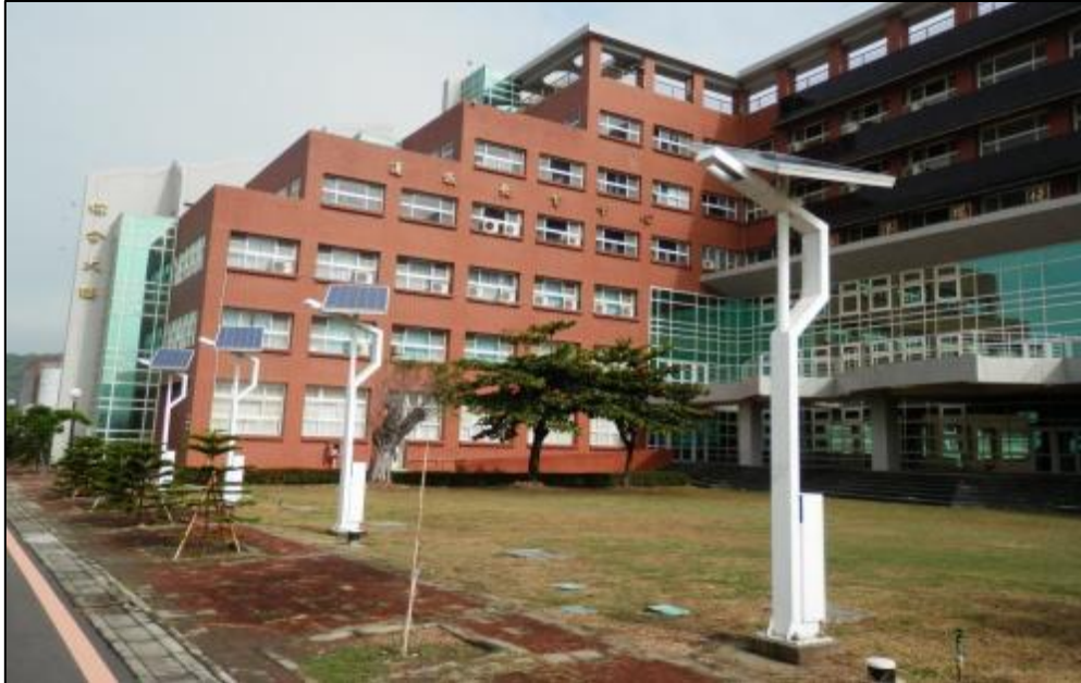
Figure 30: Solar powered lamp post in Chung San University, Kaohsiung.
