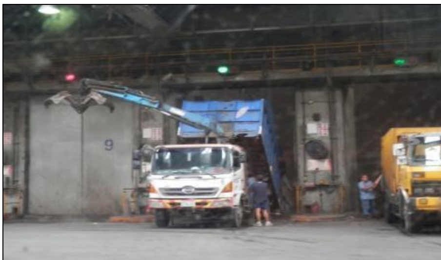
Figure 11: Garbage truck unloading waste into refuse bunker.
