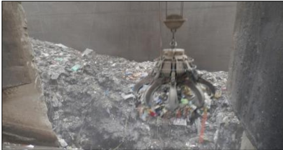
Figure 13: Refuse Crane Lifter
