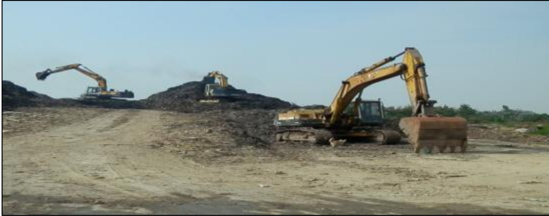
Figure 35: Part of closed Xiqingpu Sanitary Landfill that is re-excavated.
