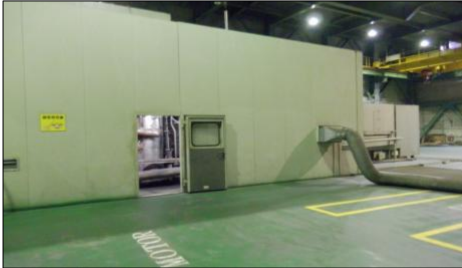
Figure 17: Condensing type turbine generator
