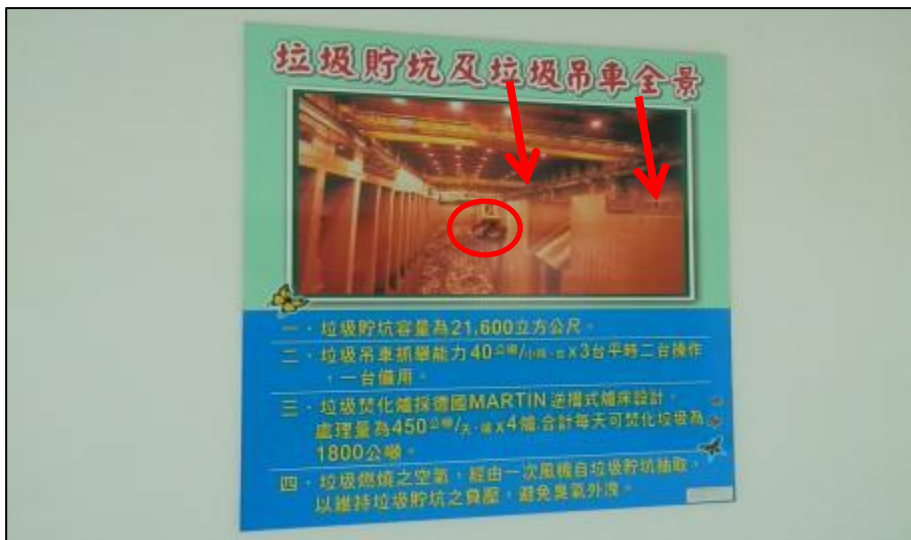
Figure 14: Refuse Crane Lifter pick up waste and feed into the stoker
