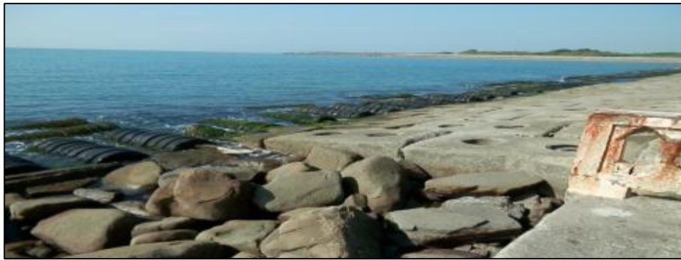
Figure 28: Unwanted tyres are being used to protect the coastline.
