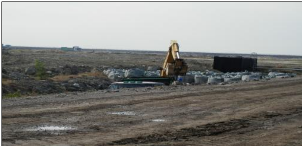
Figure 26: Land reclamation by solidified fly ash in phase 2 of the project.
