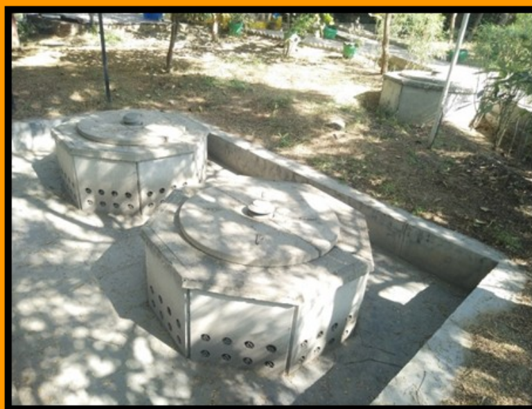
Rainwater harvesting system in one of JK Lakshmi plants
