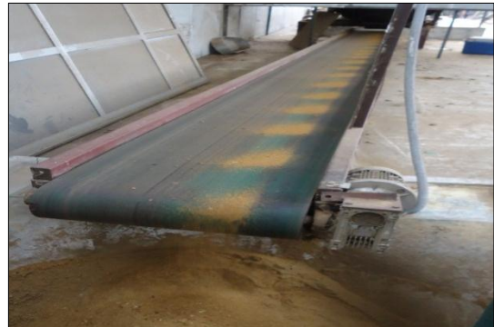
Compost processed from organic wastes
