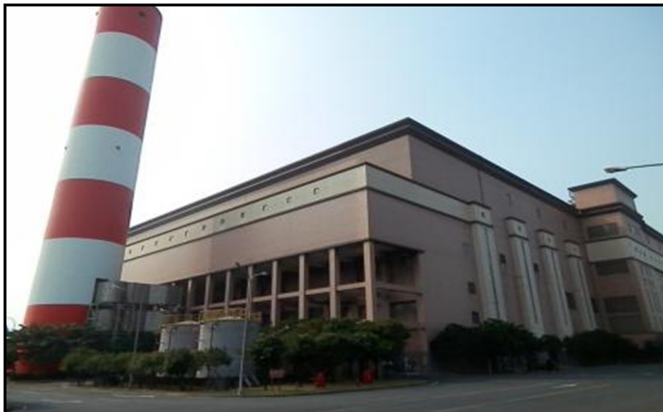
Kaohsiung City Government Environmental Protection Bureau Southern District Waste Management Plant.
