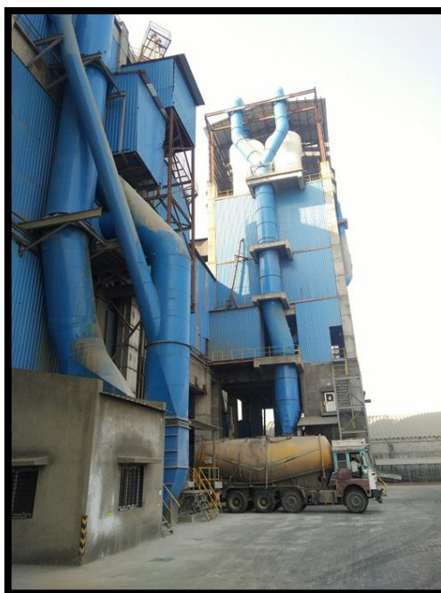
Covered channels to prevent fugitive emissions of dust
