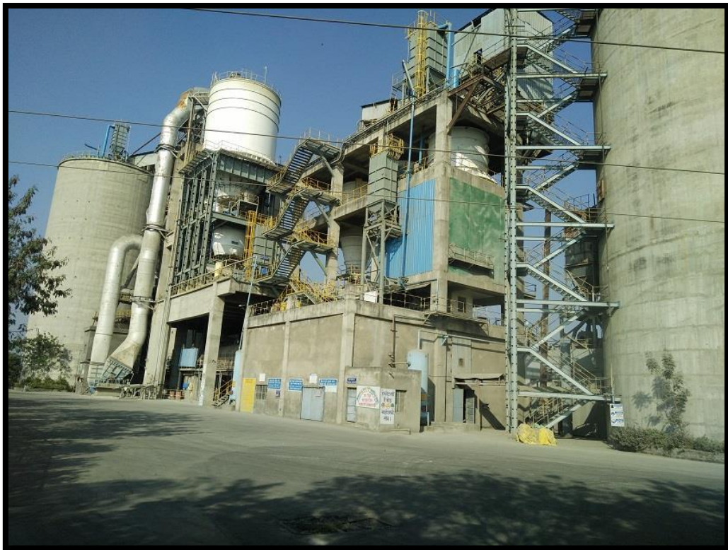
JK Lakshmi Cement -Kalol Grinding Unit, Gujarat, India
