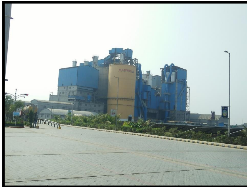
Cement grinding unit in Surat, Gujarat
