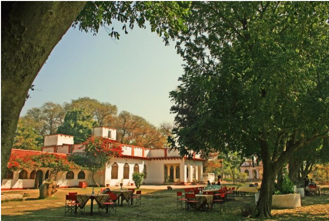
19th heritage property sensitively restored.
