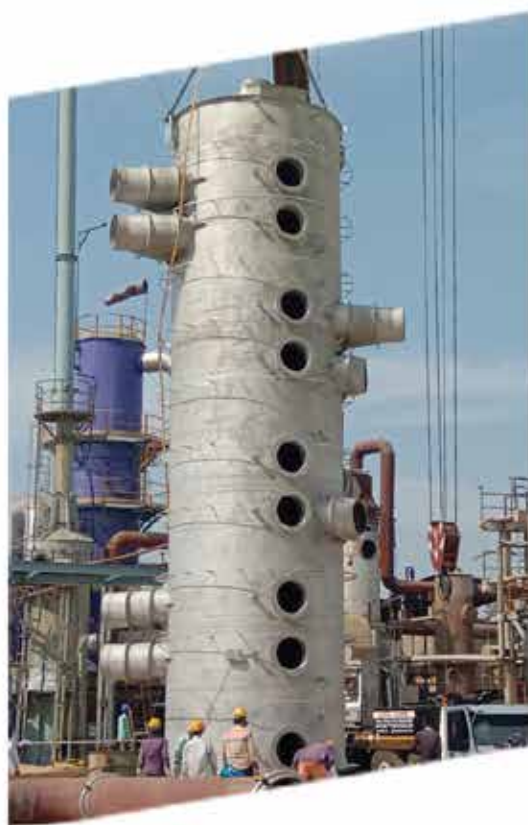
Sulphuric Acid Plant Revamped with SS304H SS Convertor, Commissioned Oct 2018
