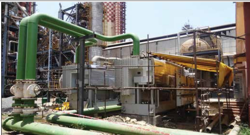
Figure 12. VAM installed in Urea Plant
