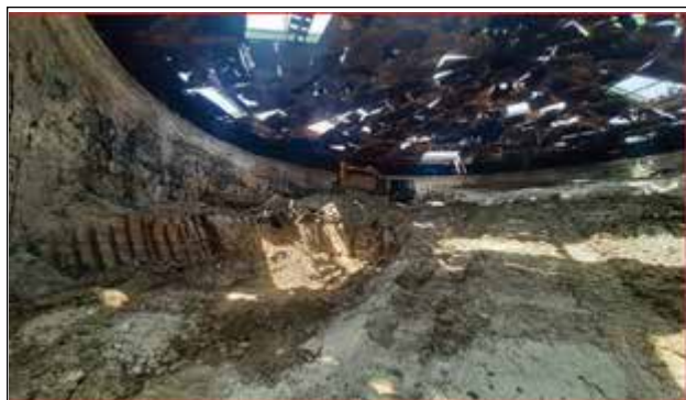
Figure 4. Cleaning of phosphoric acid tanks
