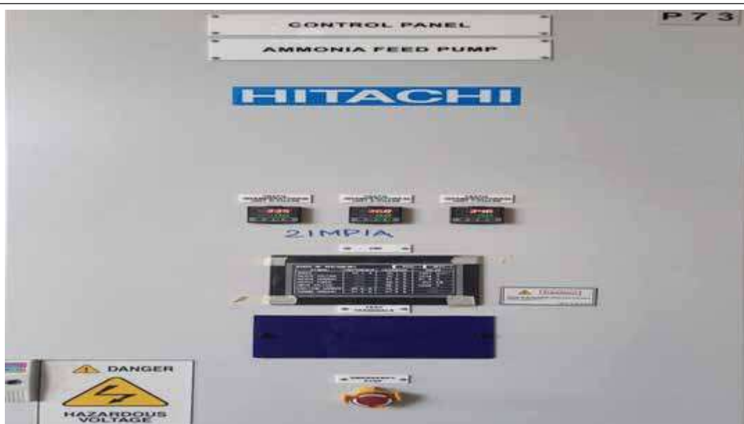
Figure 14. Control panel for P-1 pump VFD in urea plant
