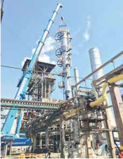
Figure 2. Saturator installation in the German plant
