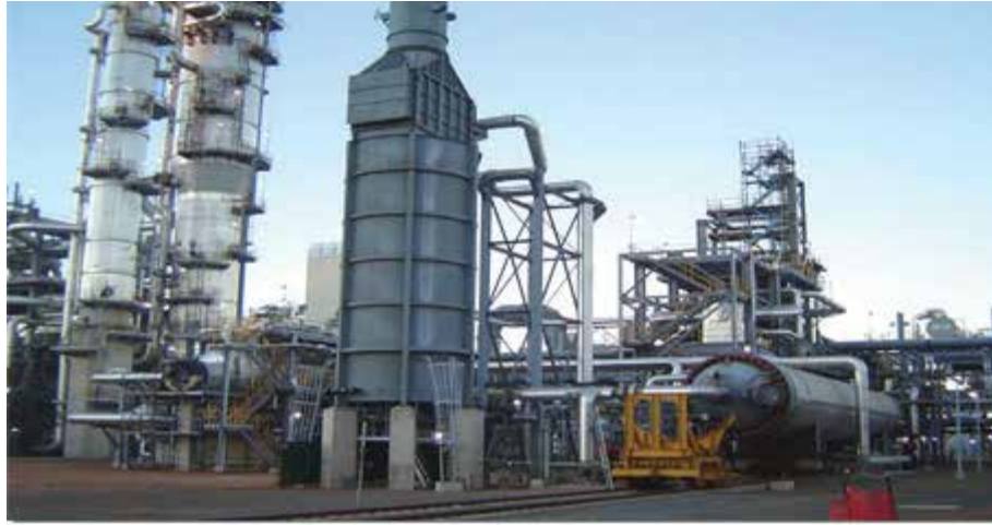
Photo 1. KBR Ammonia Synthesis Loop
